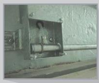
**Hidden sampling**A tiny VESDA sampling capillary is hidden behind a light fitting, invisible to unsuspecting occupants.
